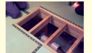
Seismic isolation devices installed in their own house. One tatami mat has been replaced with glass, enabling clients to view the installation.
