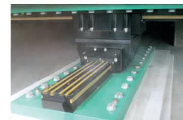
Seismic isolators installed in the foundation of the Sekigahara town office (Gifu Prefecture)
