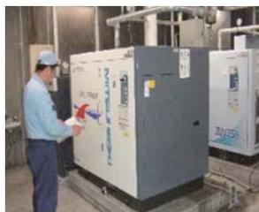
▲ Water-lubricated compressor at the YAMAGUCHI Plant
