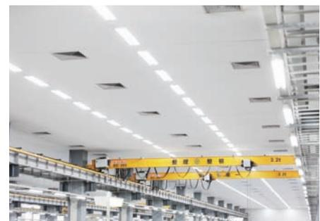
LED lights in a grinding facility. LED lighting consumes only one-third of the electricity required for mercury lights.
